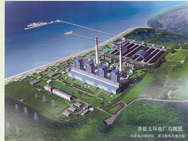
Yuhuan power plant in Zhejiang Province Ultra-supercritical 4 \times 1000\text{MW}
